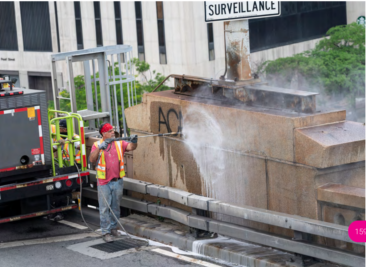
Graffiti cleaning system with pressure hoses in New York City (United States).
