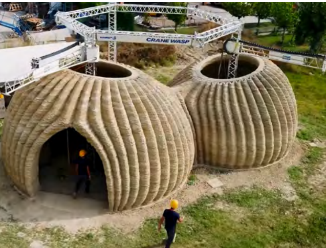
(Italy): photo of TECLA, the first structure completely 3D printed with natural materials, by WASP company.
