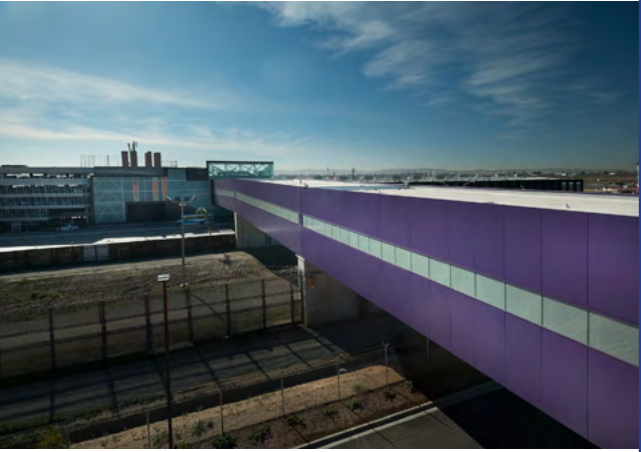
The CrossBorder Express (CBX), an international pedestrian bridge system, which charges a fee of $16 USD to access the Tijuana airport (Mexico) from a terminal in San Diego (United States).
