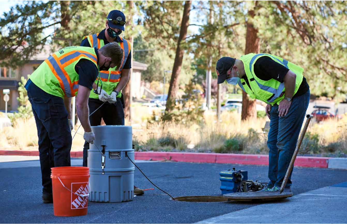
Wastewater monitoring system for the detection of COVID-19 outbreaks at universities such as Oregon State University and the University of Arizona.
