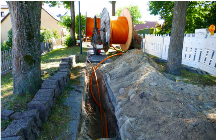
Programs for the modernization of the internet infrastructure through fiber optics.
