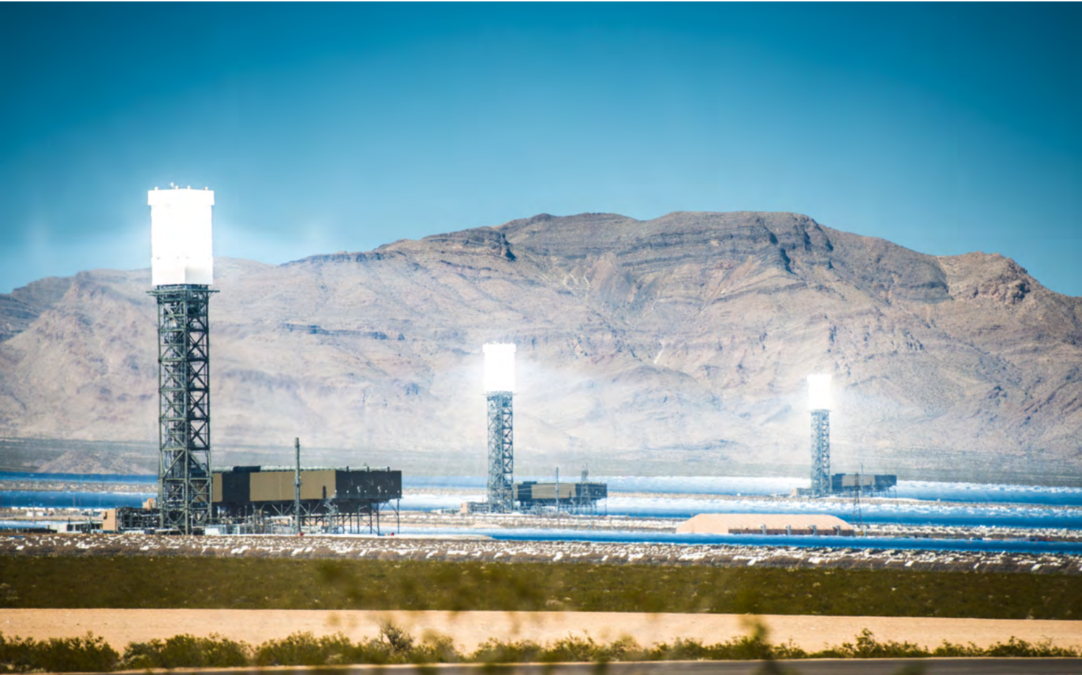
Concentrated solar thermal plant in California's Mojave desert (United States).
