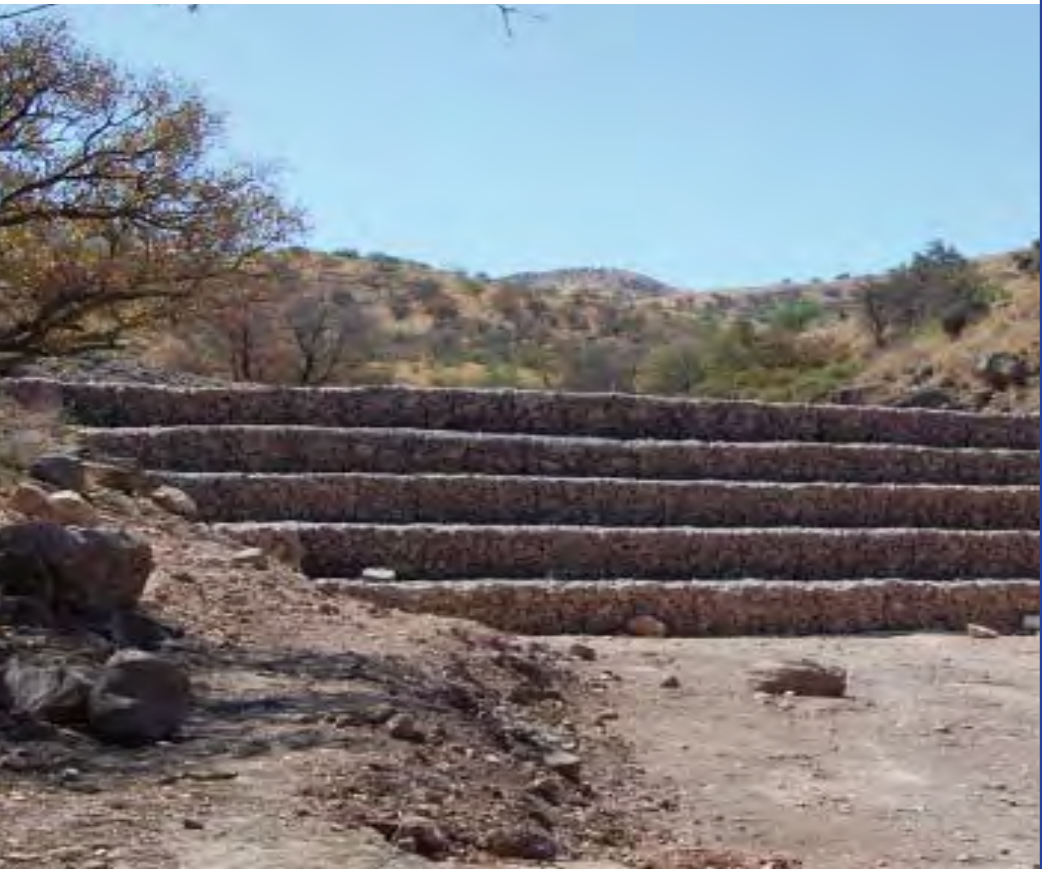
One of 18 rainwater harvesting dams designed in 2008 to hold rainwater during the first 30 minutes of rainfall as a strategic solution to the disasters caused by rainfall each year in the city of Nogales, Mexico.
