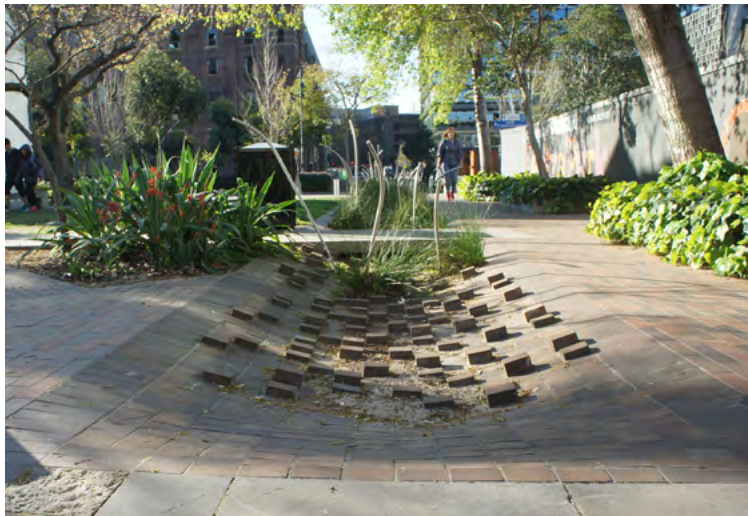
Green infrastructure systems for rainwater harvesting at Balfour Park in Chippendale (Australia).
