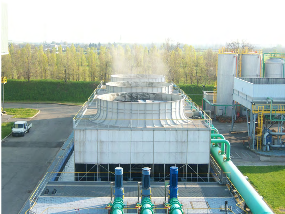
Waste-to-energy plant in Brescia, Italy.
