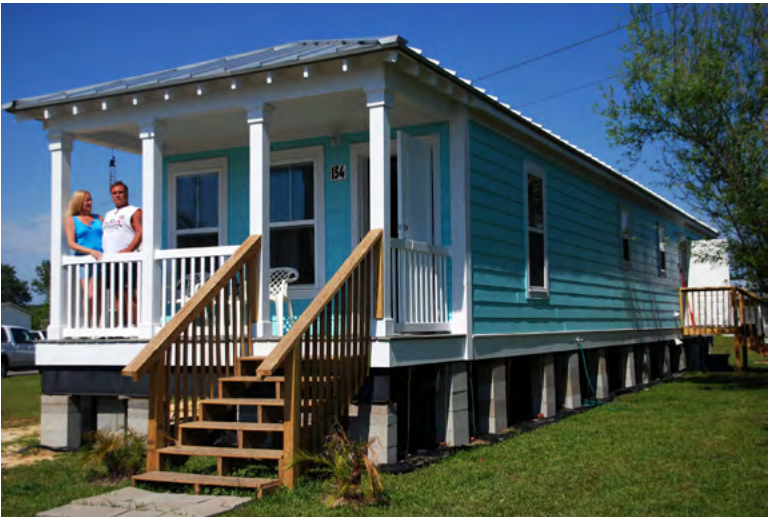
Housing program, designed by Marianne Cusato, with new urbanism principles, as part of the program for families affected by Hurricane Katrina in 2005, with which the U.S. Federal Emergency Management Agency (FEMA) has managed to house more than 2,800 families.
